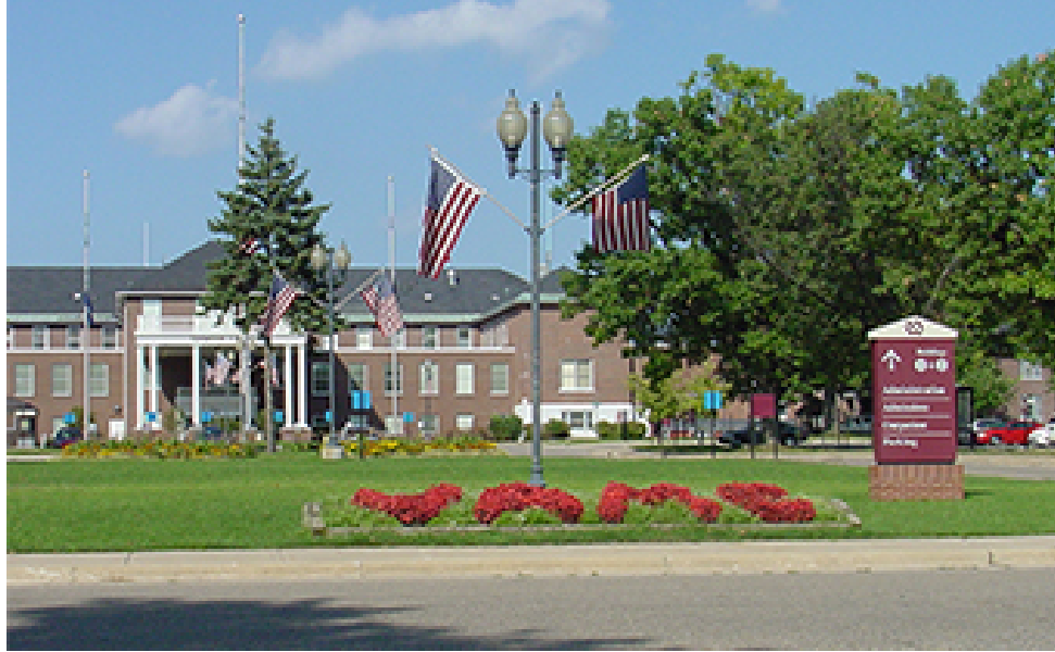
Figure 2.2 Battle Creek VAMC (Main Building) Source: Veterans' Administration (2014)
